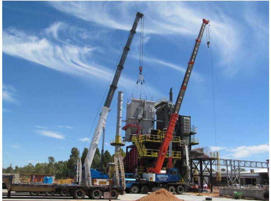
Fitting in place the post-combustion and inversion chamber
