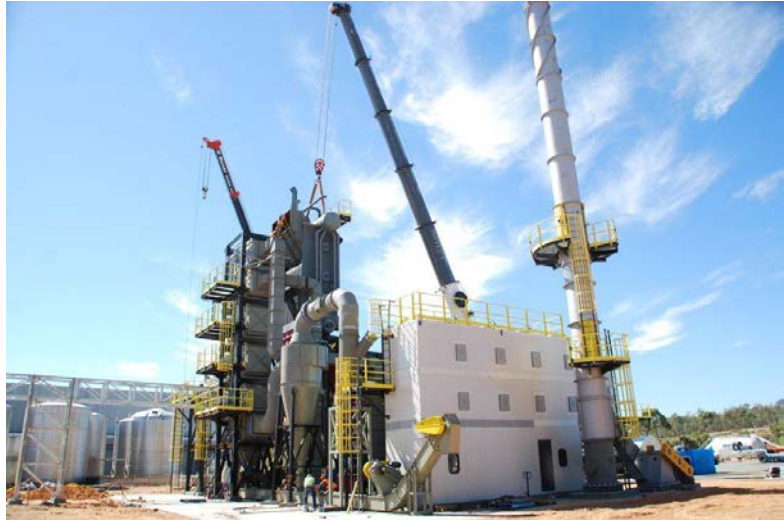
Positioning of the post-combustion and inversion chamber, with the two-drums evaporator already installed.
