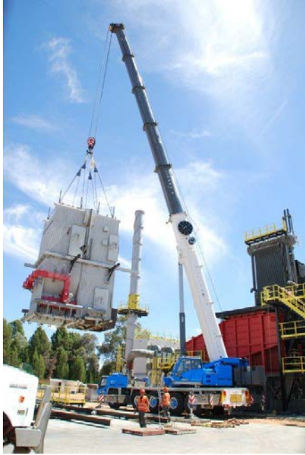
Positioning of the post-combustion and inversion chamber, with the two-drums evaporator already installed.
