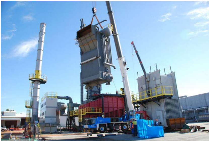
The 35-ton two-drums evaporator is lifted by a 400-tons crane
