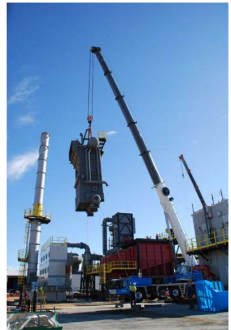
Fitting in place the post-combustion and inversion chamber
