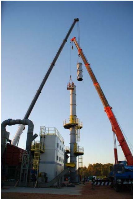
Stack assembly, up to 25 meter
